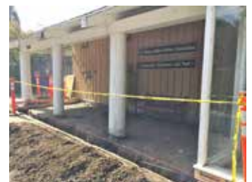
Footings are dug for the many-windowed porch library.
